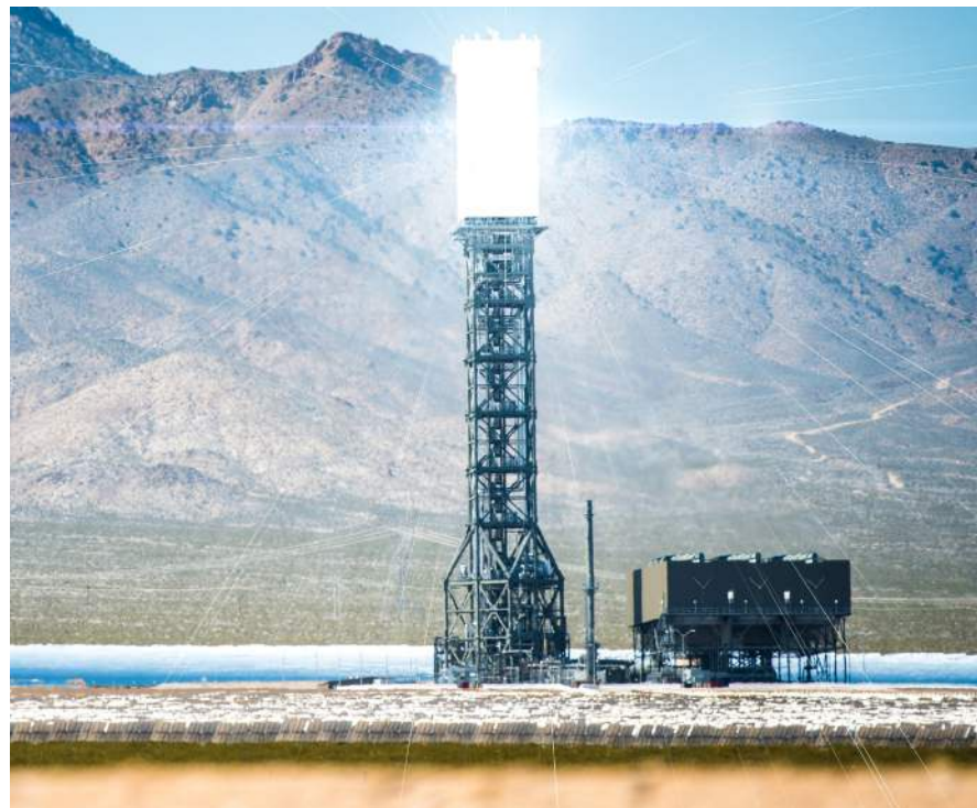
Mirrors redirect solar rays to heat the giant thermal boiler.
